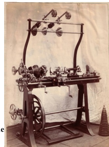
High class Ornamental Turning Lathe by Birch c. 1890
